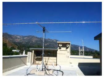
**CubeSat Tracking Station** UHF/VHF (receive-only) and other capabilities
