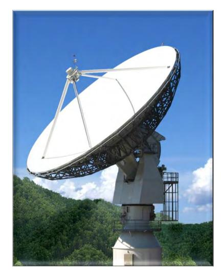
•Full-Motion, High Precision Dish Designed and Built with NASA assistance •Operational in 2006 Replaceable feeds including L-band, S-band, C-band, and Ku-band •Provides Experimental and IOAG Compatible **TT&C** Services •Operated Largely by Cost-effective **Undergraduate Students** •High Gain and Extreme Accuracy reduce comms link with small, low power, distant S/C •Station is ideal for LEO and lunar spacecraft experiments and operations
