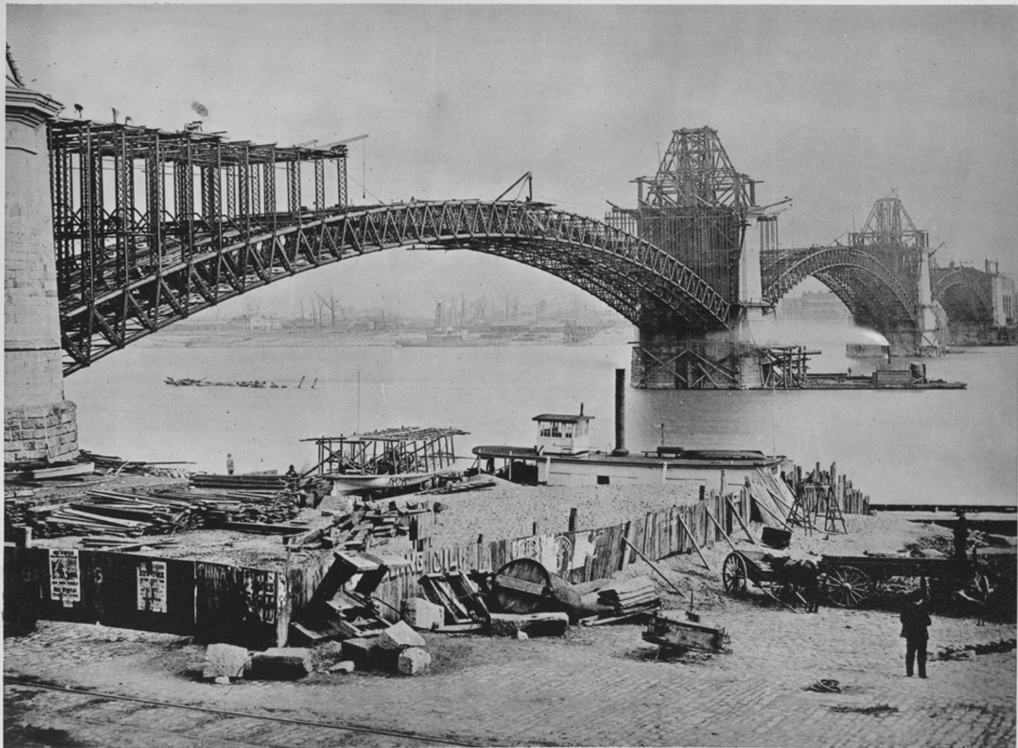
THE ERECTION. THE RIBS COMPLETED AND THE ROADWAYS BEGUN.
