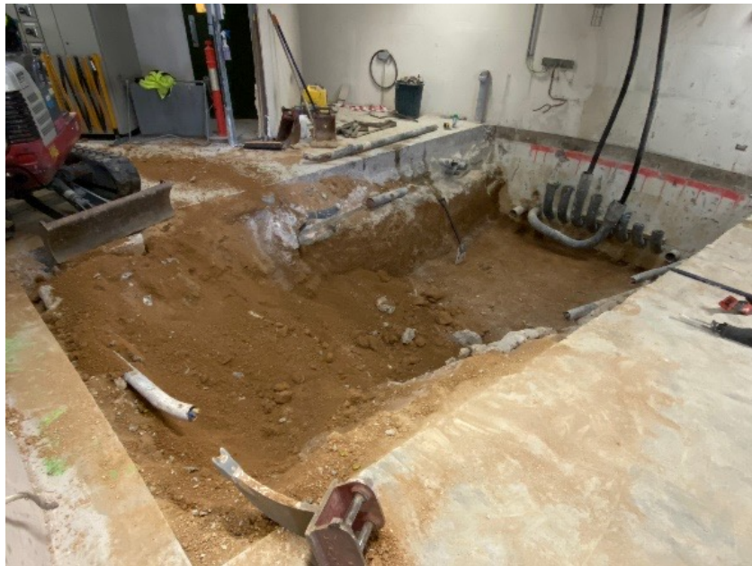
Trench Excavation for Substation
