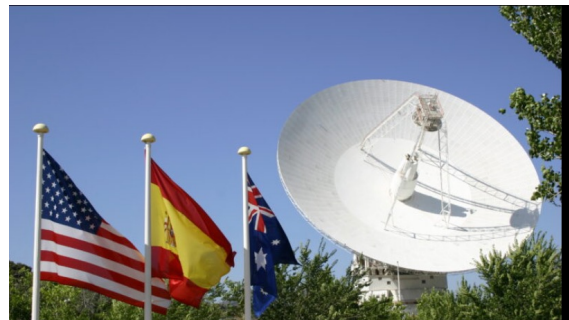
European Demonstrations Madrid DSS-63 (DSN) 70 m antenna, 20 kW transmitter, 4 cm wavelength (C band) + Medicina Antenna
