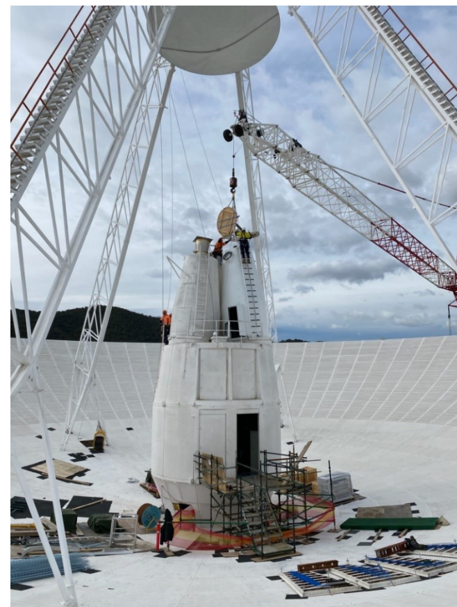
Canberra TT&C Cone Replacement
