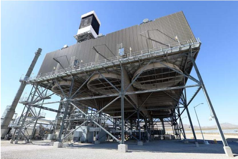
An air-cooled condenser housing giant fans
