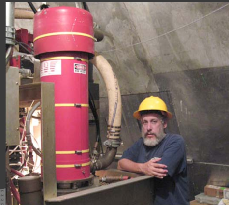
Klystron Tube; astronomer for scale
