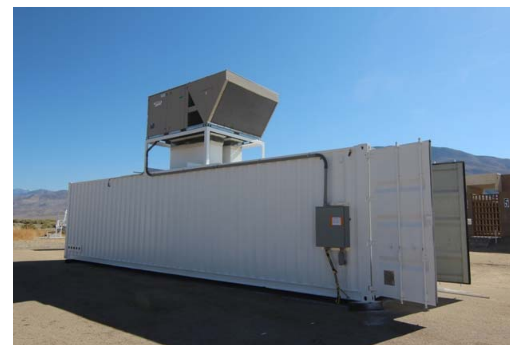
Fig. 7: The Owens Valley LWA electronics shelter, capable of supporting 50 kW of back-end electronics, including the LEDA correlator and the transient detection backend (Pulsing Planet Finder) developed at Caltech and JPL - 160 CPUs, 20 GPUs, 1 TB RAM, 200 TB Lustre storage.
