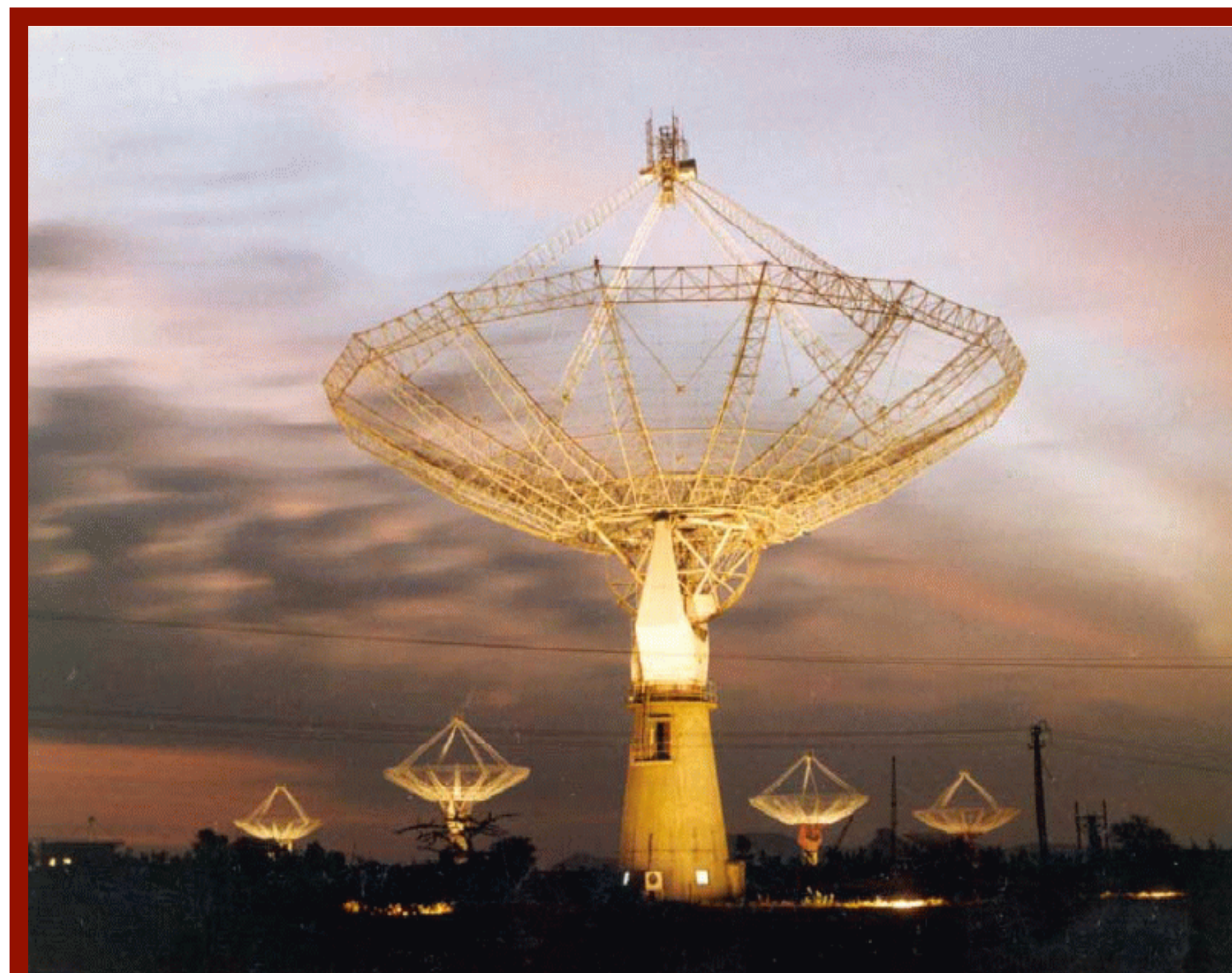
THE OBSERVATORY: The Giant Meterwave Radio Telescope (GMRT) is the largest fully steerable telescope operating at meter wavelengths. Currently, its lowest operating frequency is 150 MHz. The facility, located near Pune, India, consists of 30 individual 45 meter dishes.
