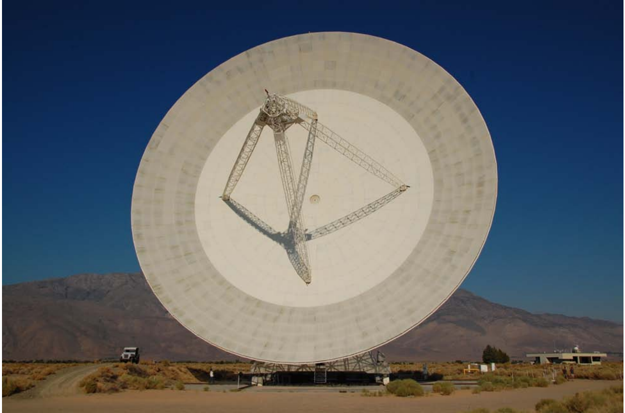
Figure 5.1: The OVRO 40 m telescope. It is a prime-focus telescope dedicated to monitoring the flux density of a large sample of blazars and other radio sources at 15 GHz.
